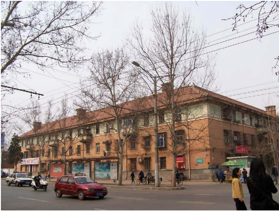
1950's worker's residential block
